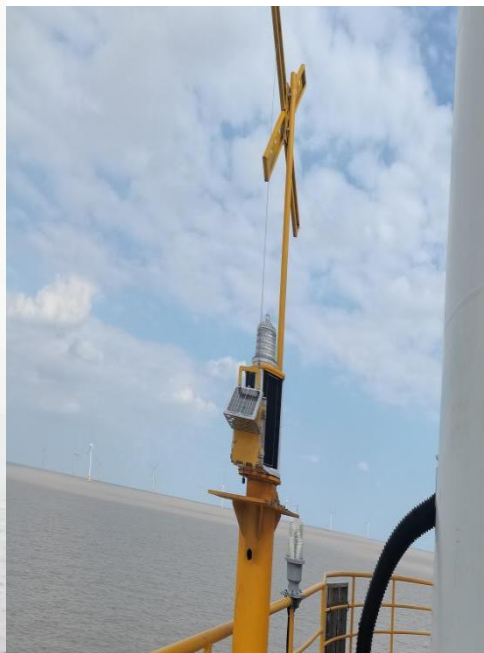
Figure 5-7 close light pile and AIS
