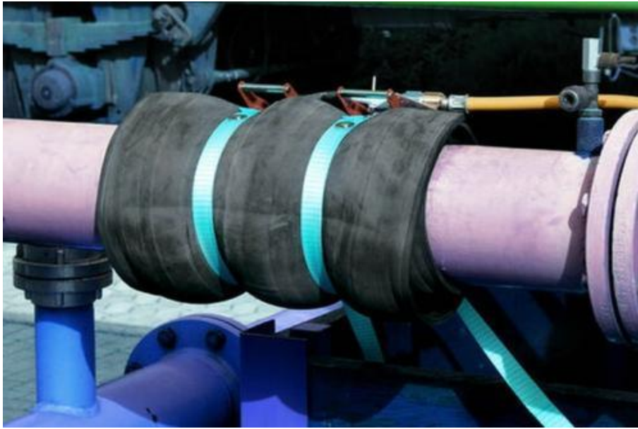
Figure 3-4 schematic diagram of plugging strip
