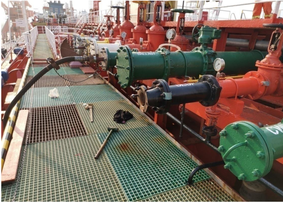
Fig. 4-1 connect nitrogen to "Guang Hui 616" main pipeline
