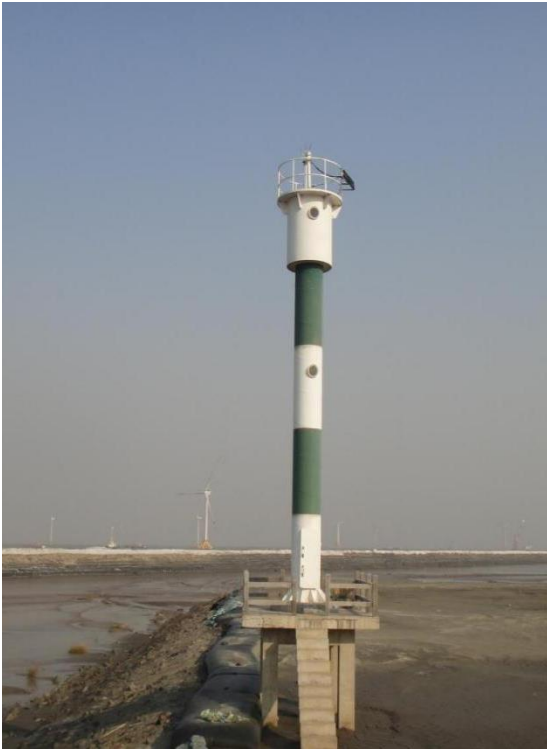
Original condition of right light pile at Liubu Port
