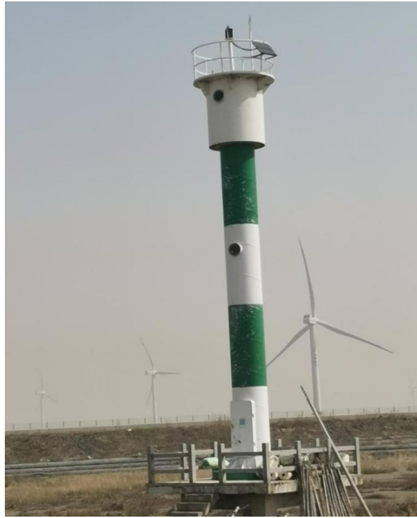
Status quo of right light pile in Liubu Port
